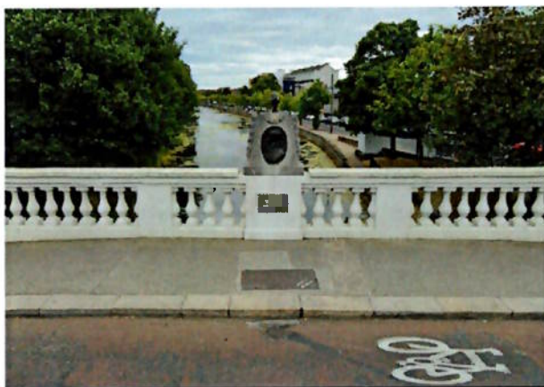
Figure 7. Robert Emmett Memorial on bridge. Under the proposed scheme design, people wishing to view the memorial will have to enter the carriageway and stand in a cycle lane, creating a safety issue.
